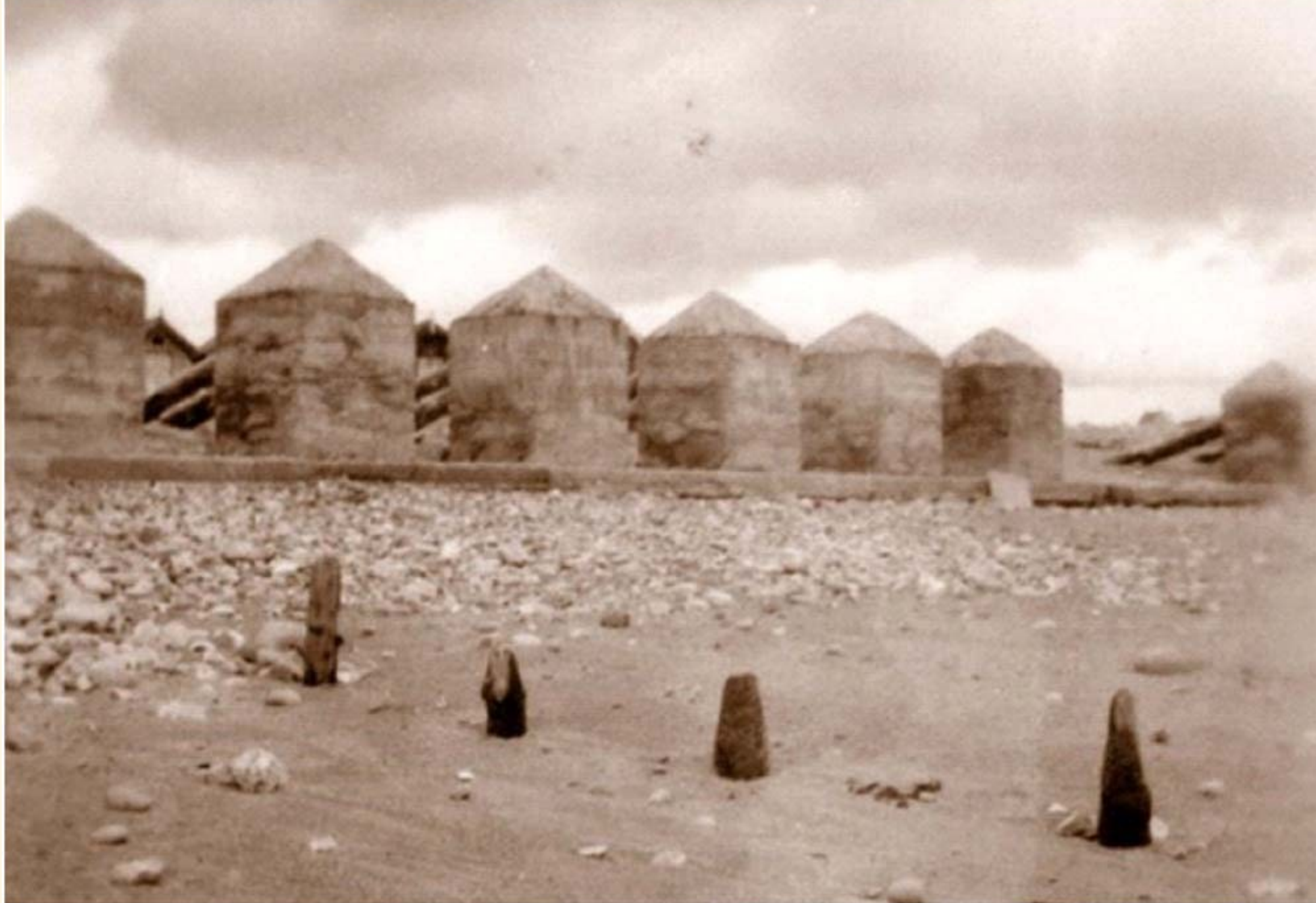
A line of concrete Dragon's Teeth along the beach. The purpose was to create obstacles if the Germans landed; these would prevent their tanks from advancing up to the village and controlling the London to Plymouth road.
